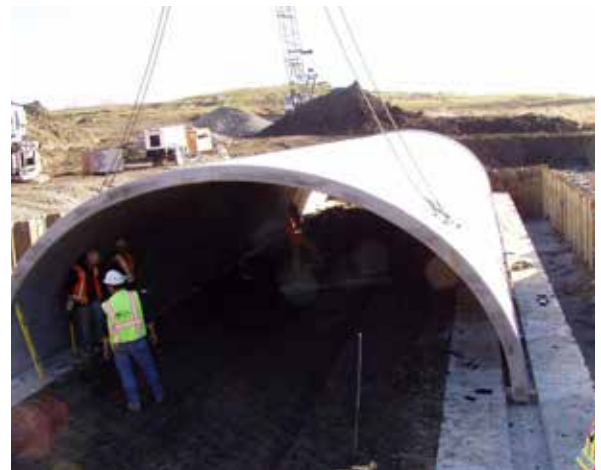
QUEENSVILLE (HWY 404 EXTENSION), ON - BEBO CONCRETE ARCH
