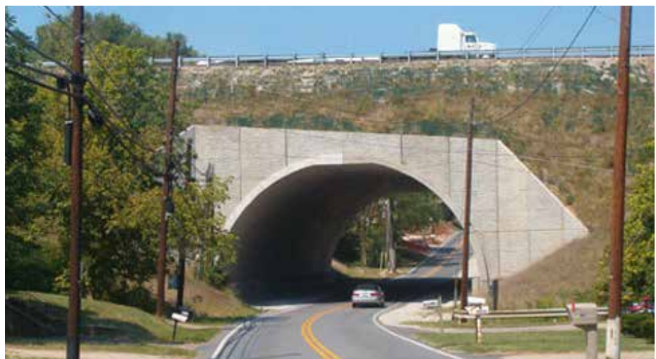
CROSSROADS, WV - BEBO CONCRETE ARCH TYPE C54T
