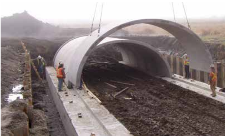
QUEENSVILLE (HWY 404 EXTENSION), ON - BEBO CONCRETE ARCH
